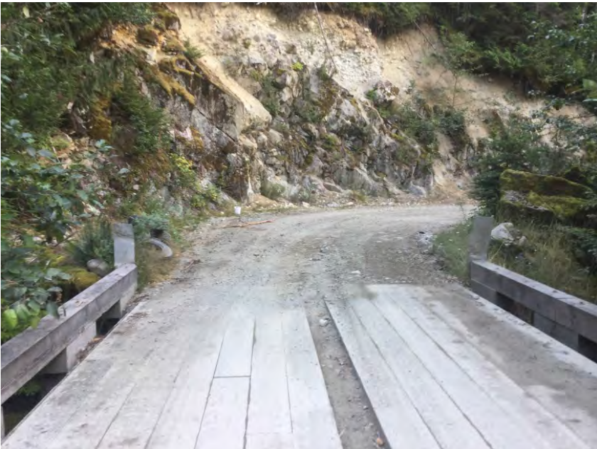
Left Approach Facing Away From Bridge
