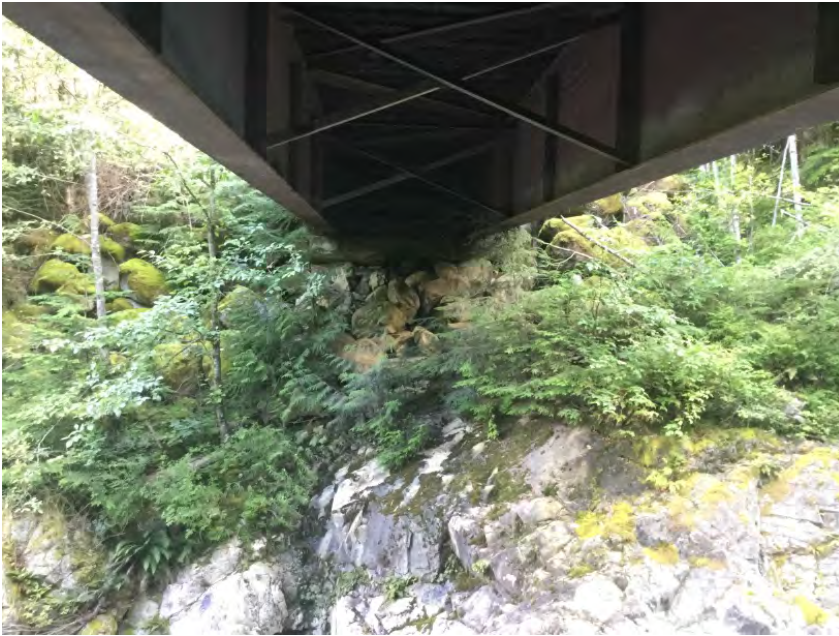
Right Bank Abutment
