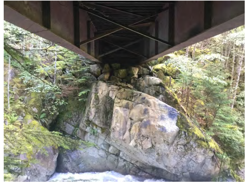
Left Bank Abutment
