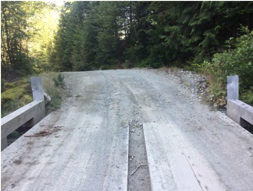
Right Approach Facing Away From Bridge
