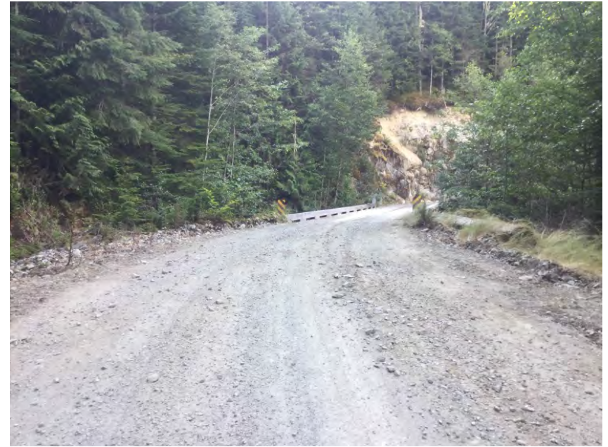
Right Approach Facing Bridge
