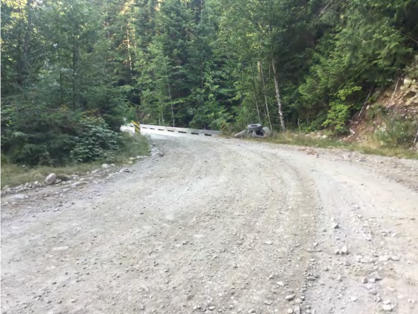
Left Approach Facing Bridge
