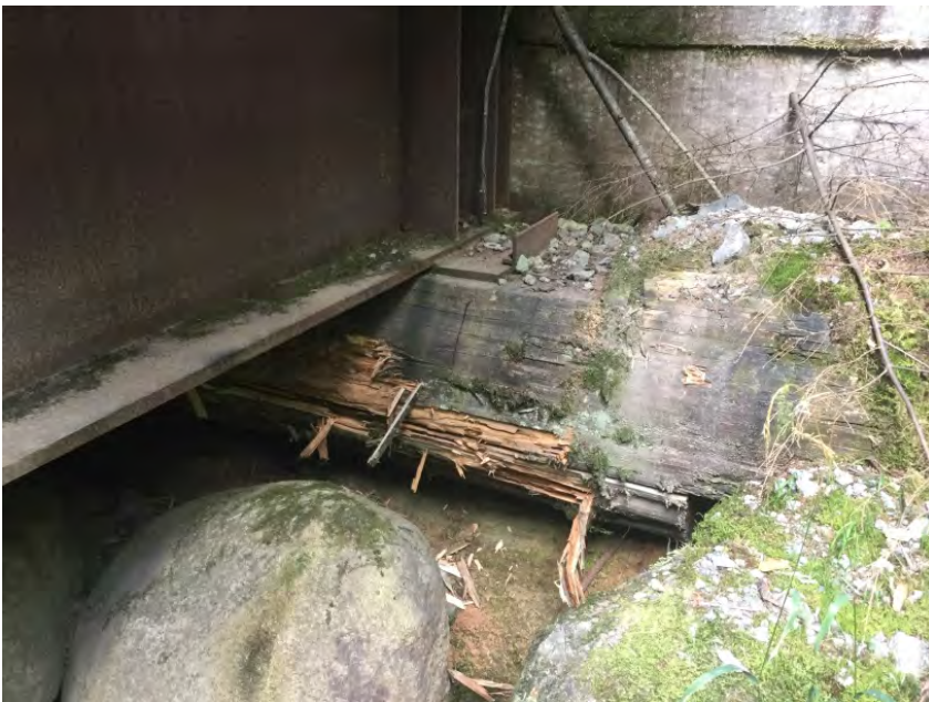
Right Abutment Upstream Corner
