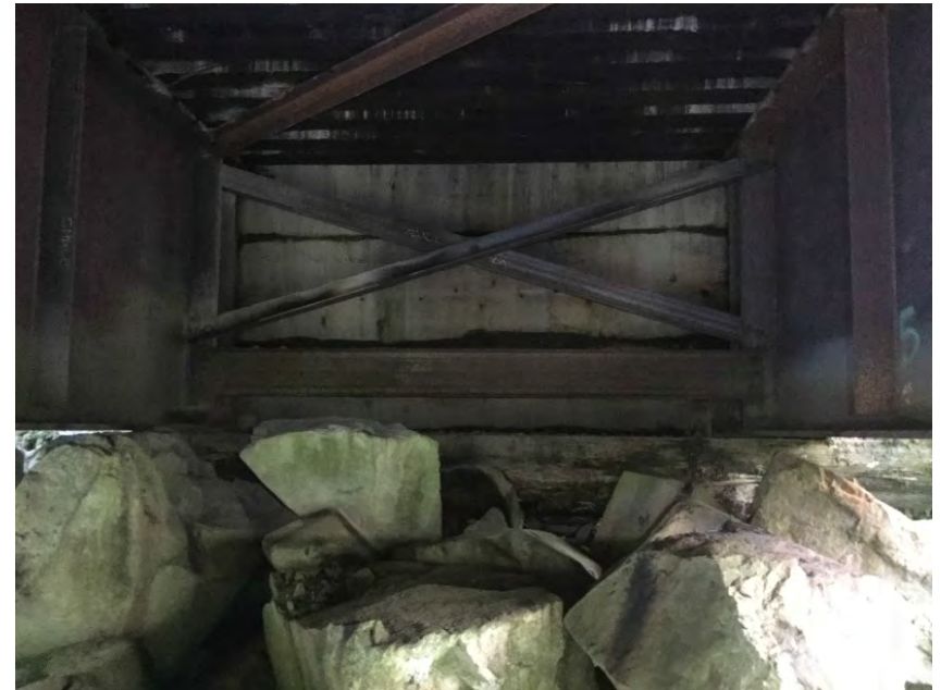
Left Bank Abutment
