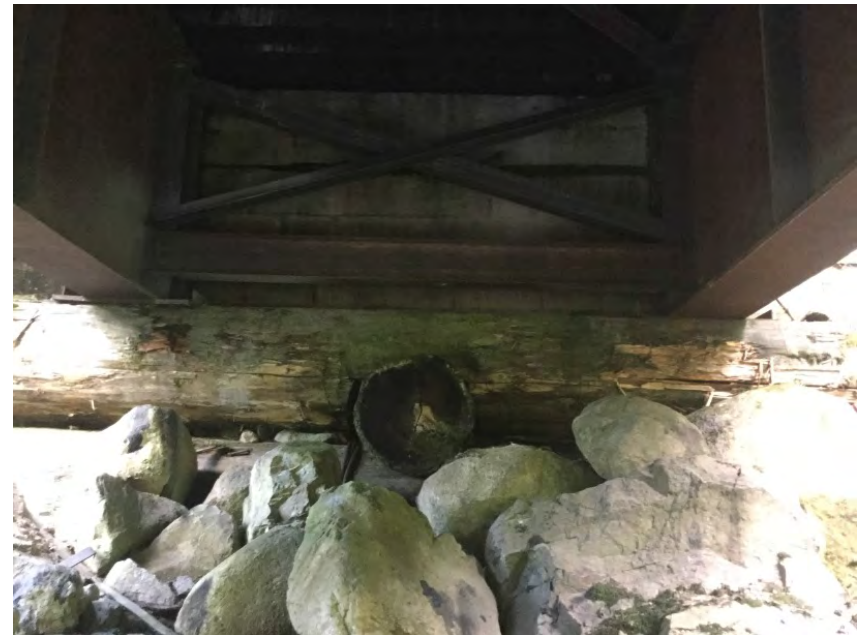
Right Bank Abutment
